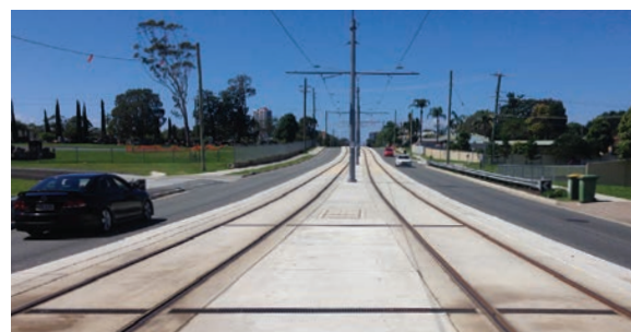
Gold Coast QLD Light Rail Project.
